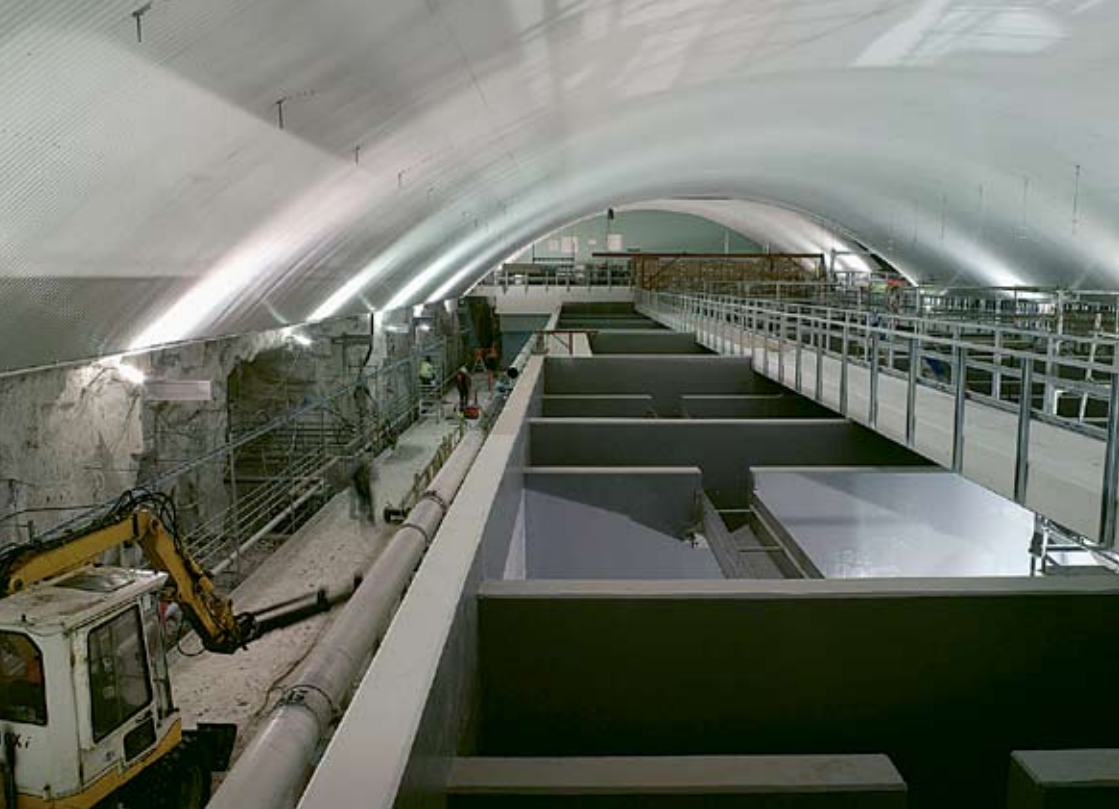
The new Oset water treatment plant under construction.
